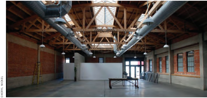
Three unused warehouses were transformed into 33 low-cost artist studio spaces and five live/work spaces in downtown San Diego's East Village (left). In July 2010, Space 4 Art opened with a huge street party, celebrating a successful community partnership of 95 percent donated time and materials and 100 percent occupancy (far left).
